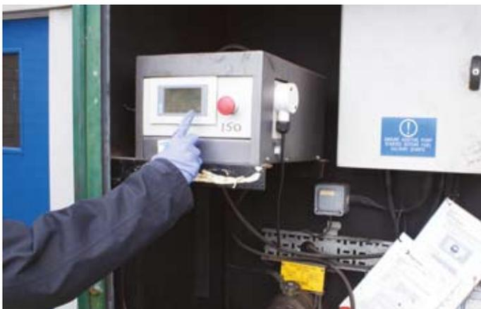
Dosing units add the correct quantity of Envirox to bulk fuel deliveries.
